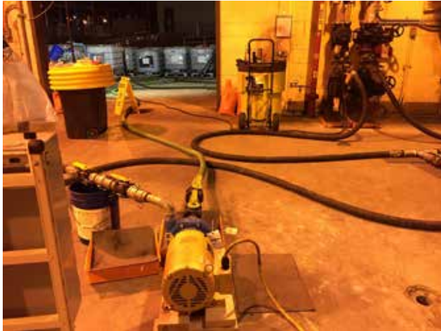
The team let the struvite dissolver soak in the pipes, agitated and recirculated it, then rinsed it out. Pumping pressure and flow rates returned to optimum levels after treatment.
