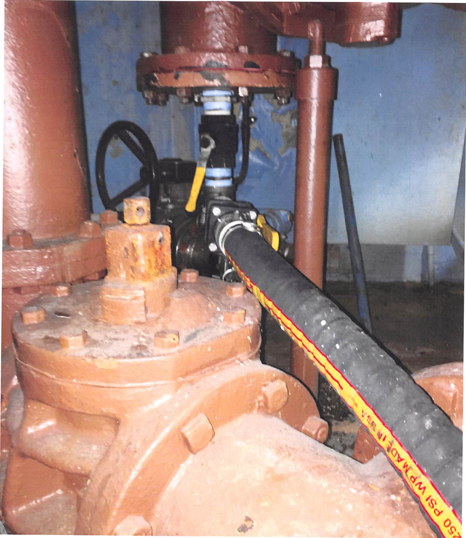
The chemical-based process for removing struvite in pipe has been successful for the Bethlehem Wastewater Treatment Plant's internal distribution lines.
